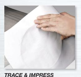
Trace pipe's inner diameter. Create an impression of the pipe. Fold to form 90° angle.
