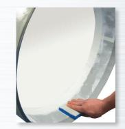
The dampened sponge will reactivate the adhesive to ensure zero air permeability.
